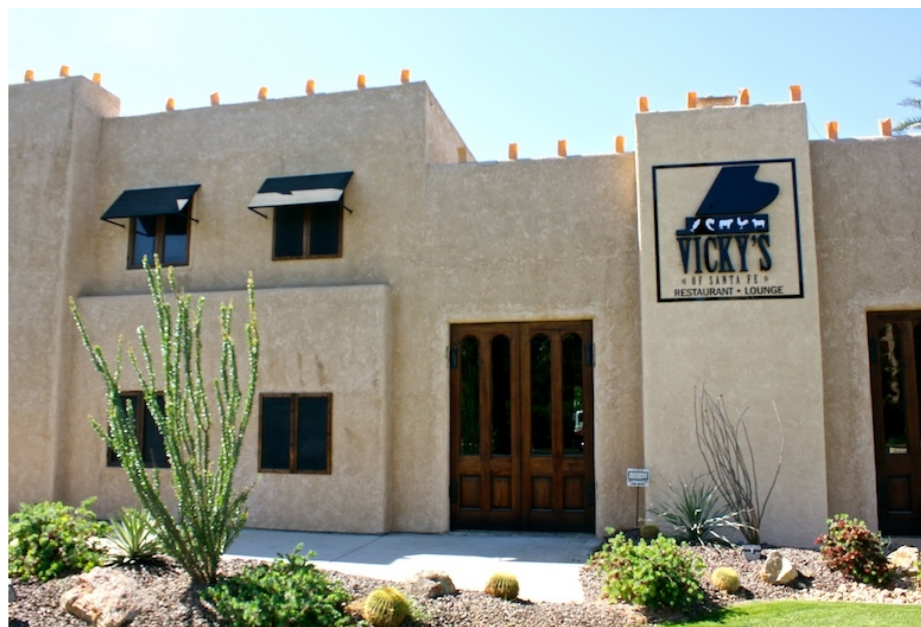
Vicky's of Santa Fe in Indian Wells was built in 1989 and originally was to be named Vanessa's of Santa Fe.
